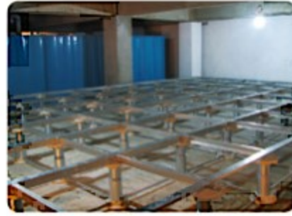
Assembling Skid Base & Leveling
